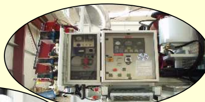
Control panel located outside the danger zone (or pressurized in a danger zone)
